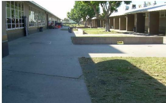
Overall paving in poor condition across campus.
