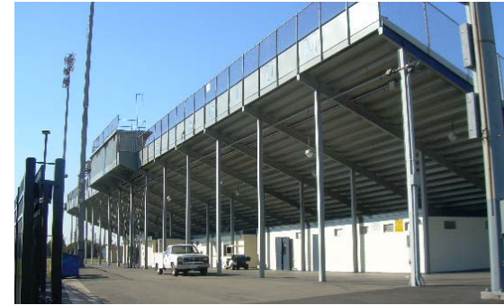
Stadium is in need of renovation
