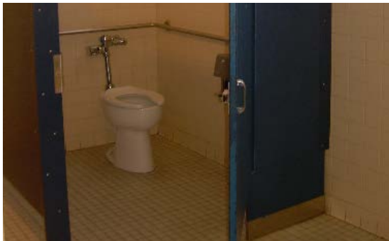
Upgrade and expand restroom facilities.
